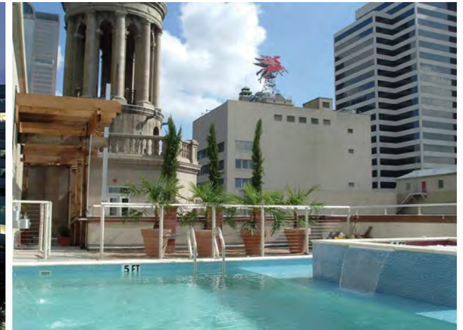
Davis Building, Dallas
